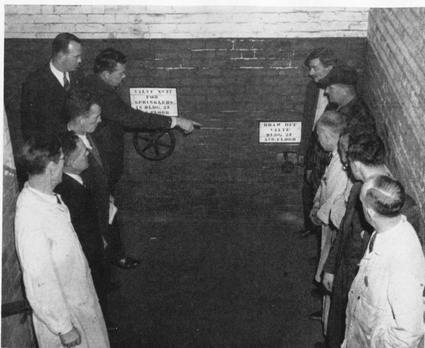
This emergency crew from the first and second shifts of Fuse Loading are receiving instructions from Fire Inspector Herman Hansen on the functioning of the sprinkler shut off valve and draw off valve. This same crew of men receive instruction as stretcher teams and are familiar with power controls, and check evacuation of all employees during fire drills.
